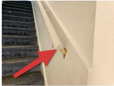
Bottom of staircase
