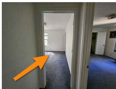
Door to upstairs bedroom at southwest corner of house
