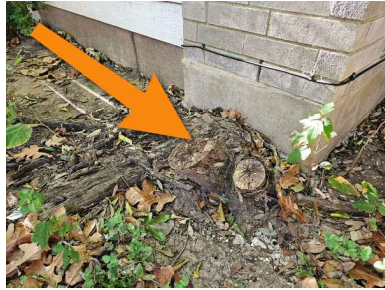
Northwest corner of house
