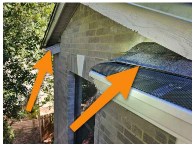
Small sections at front of house - photo
