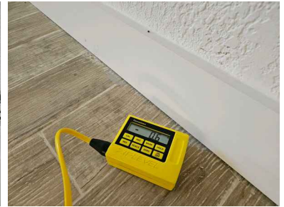
Downstairs living room at west side of house
