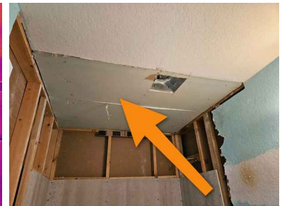
Above upstairs bathroom
