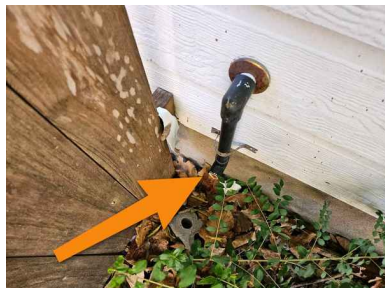
Northwest corner of house - photo 1
