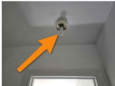
In bedroom closet at southwest corner of house
