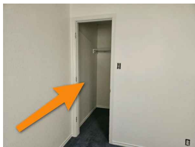
Closet door at upstairs front bedroom
