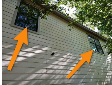
South side of house
