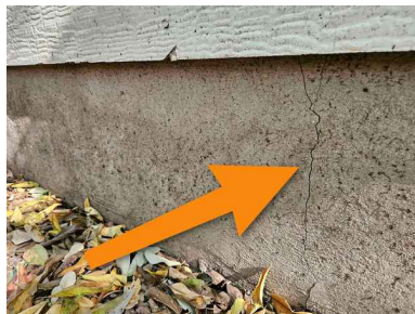
South side of house
