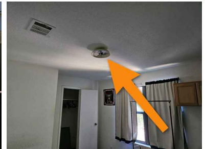
Upstairs front bedroom
