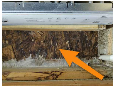
Below HVAC unit looking up
