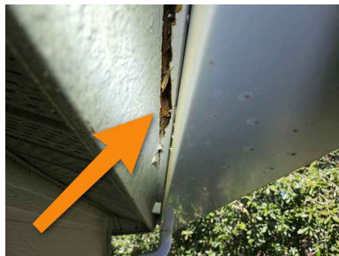
Behind gutter system at various locations at front of house
