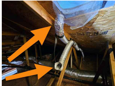
Above hallway bathroom in attic area
