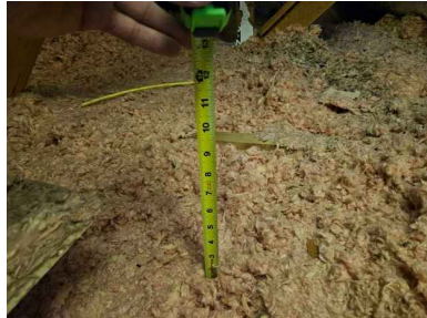
Approximately 2-4 inches of insulation present in attic area
