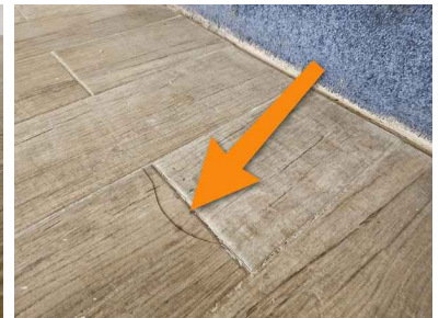
Bottom of staircase
