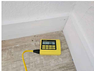
Downstairs living room at southwest corner of house
