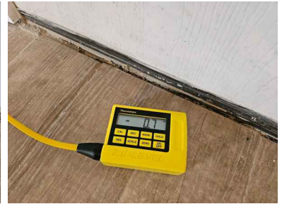
At garage door
