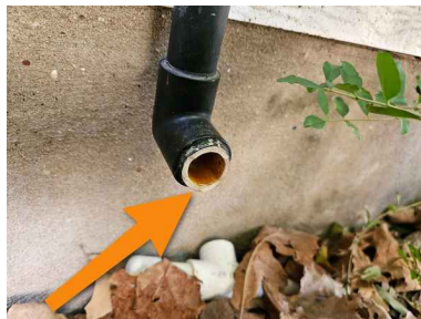
Northwest corner of house - photo 2
