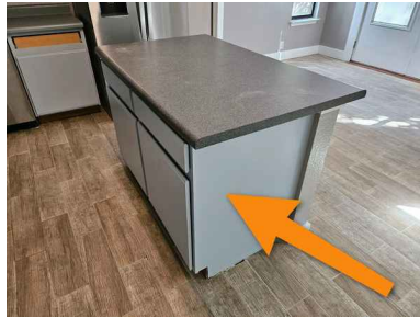
Kitchen island loosely installed
