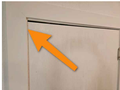
Contact at door to garage
