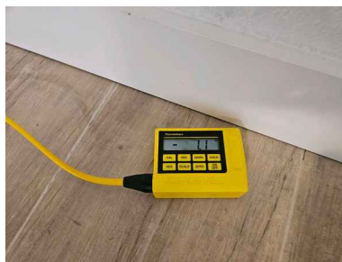
Northeast corner of house
