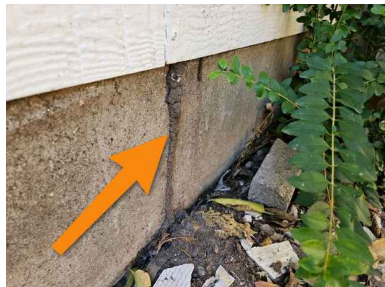
Mud tube at north side of house
