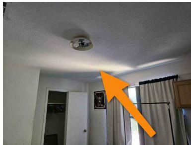
Above bedroom at northwest corner of house
