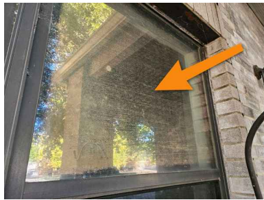
Lower window at entryway
