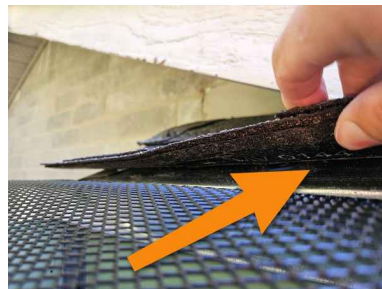
Small sections at front of house - photo
