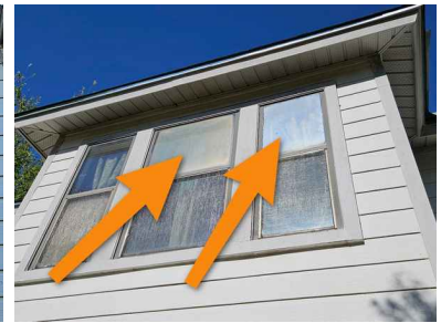
Upper windows at back of house
