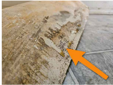
Below flooring in pantry
