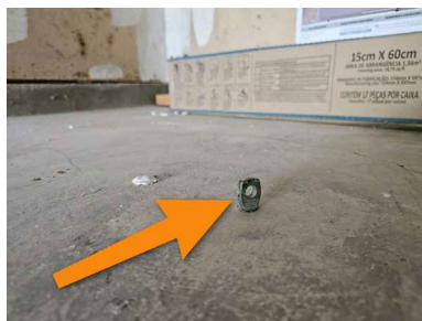
Garage near sub panel
